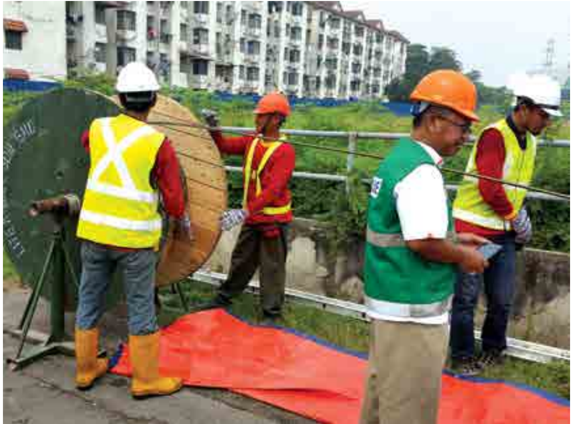
Site Inspection by OSHE Team
